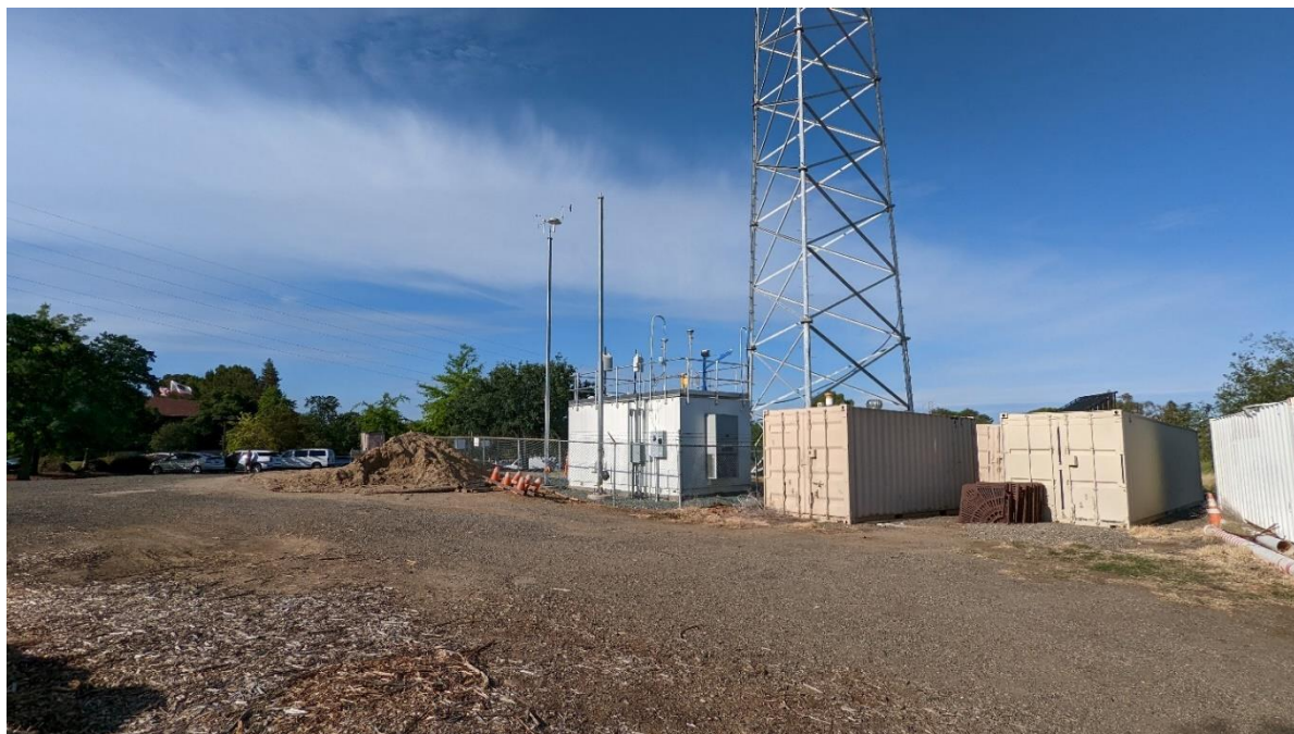
Figure 28 – Folsom-Natoma St. Site Photo
