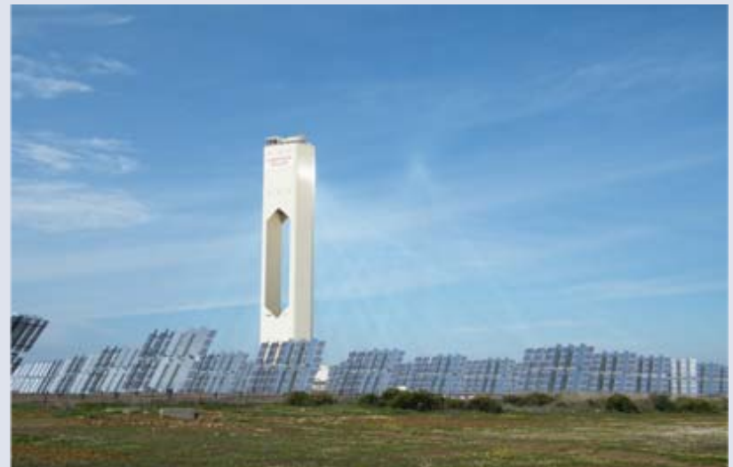
Source: Abengoa – Power Technology
