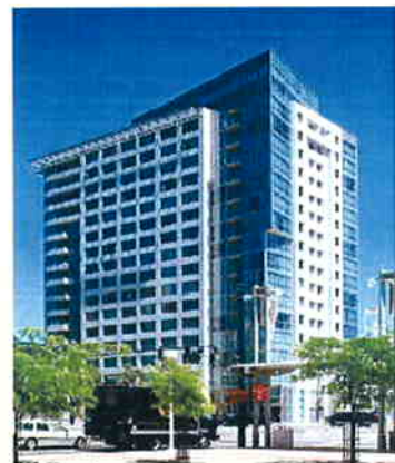
Avalon I 16-story residential San Francisco, CA Fisher Friedman, Architects
